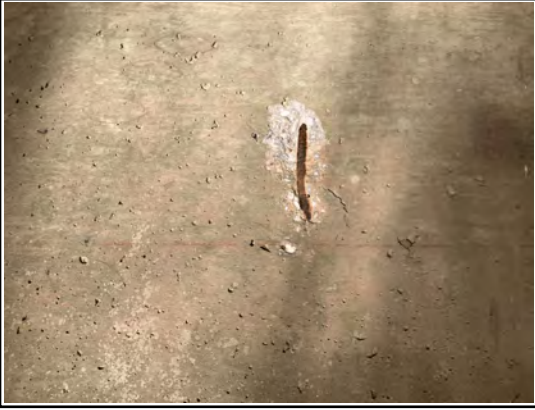
rebar span 10 girder 2
