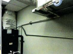
Verify unit shut down with EZ Trap float switches and pan switches. When tested, the units did not shut down.
