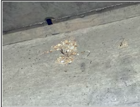
spall bent cap 3 span 3 over pile 2
