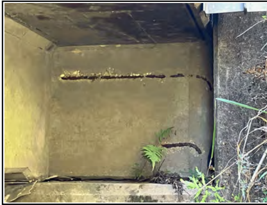
rebar at abut 1 near wing
