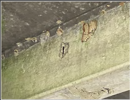
spall span 4 beam 2
