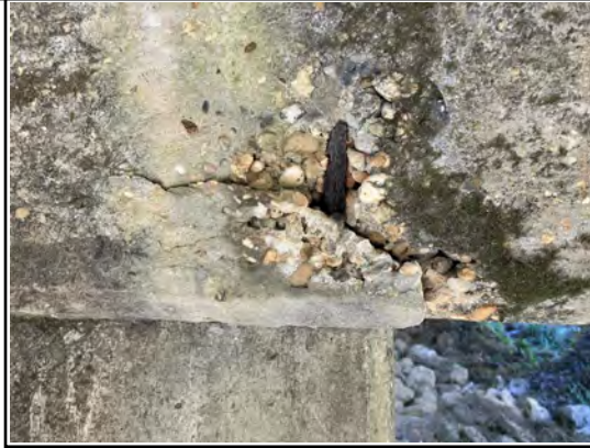
spall bent cap 3 span 3 over pile 2
