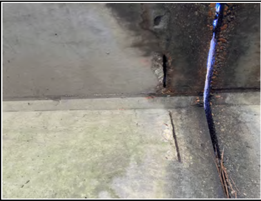
spall right overhang span 5
