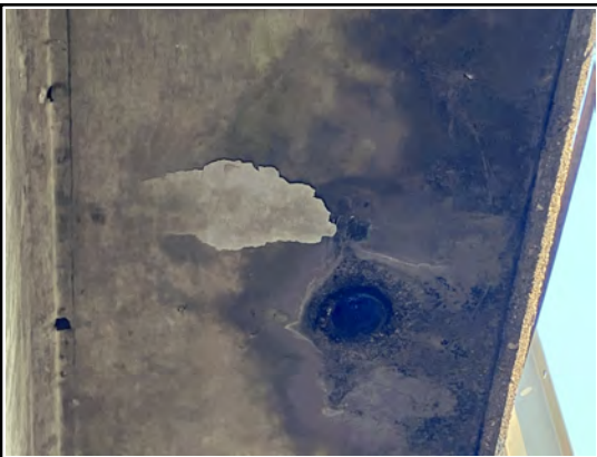
delam right overhang span 4
