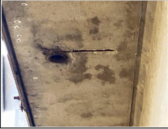
spall right overhang span 5
