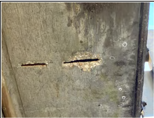
spall span 4 beam 2
