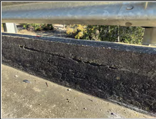
rebar right curb span 6
