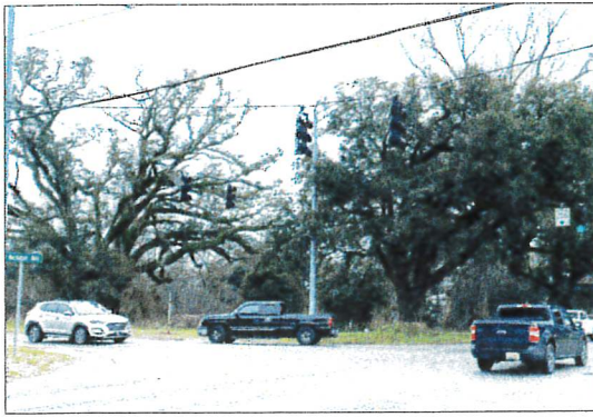
PHOTO PROVIDED Traffic moves through the intersection of South Hickory Street and West Michigan Avenue. Foley will install new signals at the site as part of plans to add turn lanes to improve the intersection.
