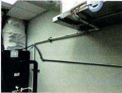
7. Verify unit shut down with EZ Trap float switches and pan switches. When tested, the units did not shut down.
