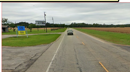
Lipscomb Rd Looking West
