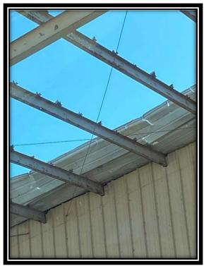
Photo No. 3 – Roof Damage from Hurricane
