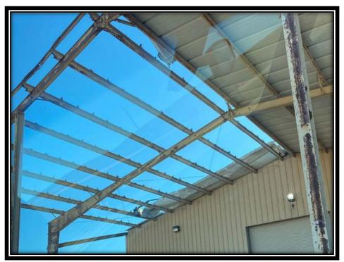
Photo No. 1 – Roof Damage from Hurricane
