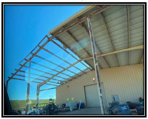
Photo No. 2 – Roof Damage from Hurricane
