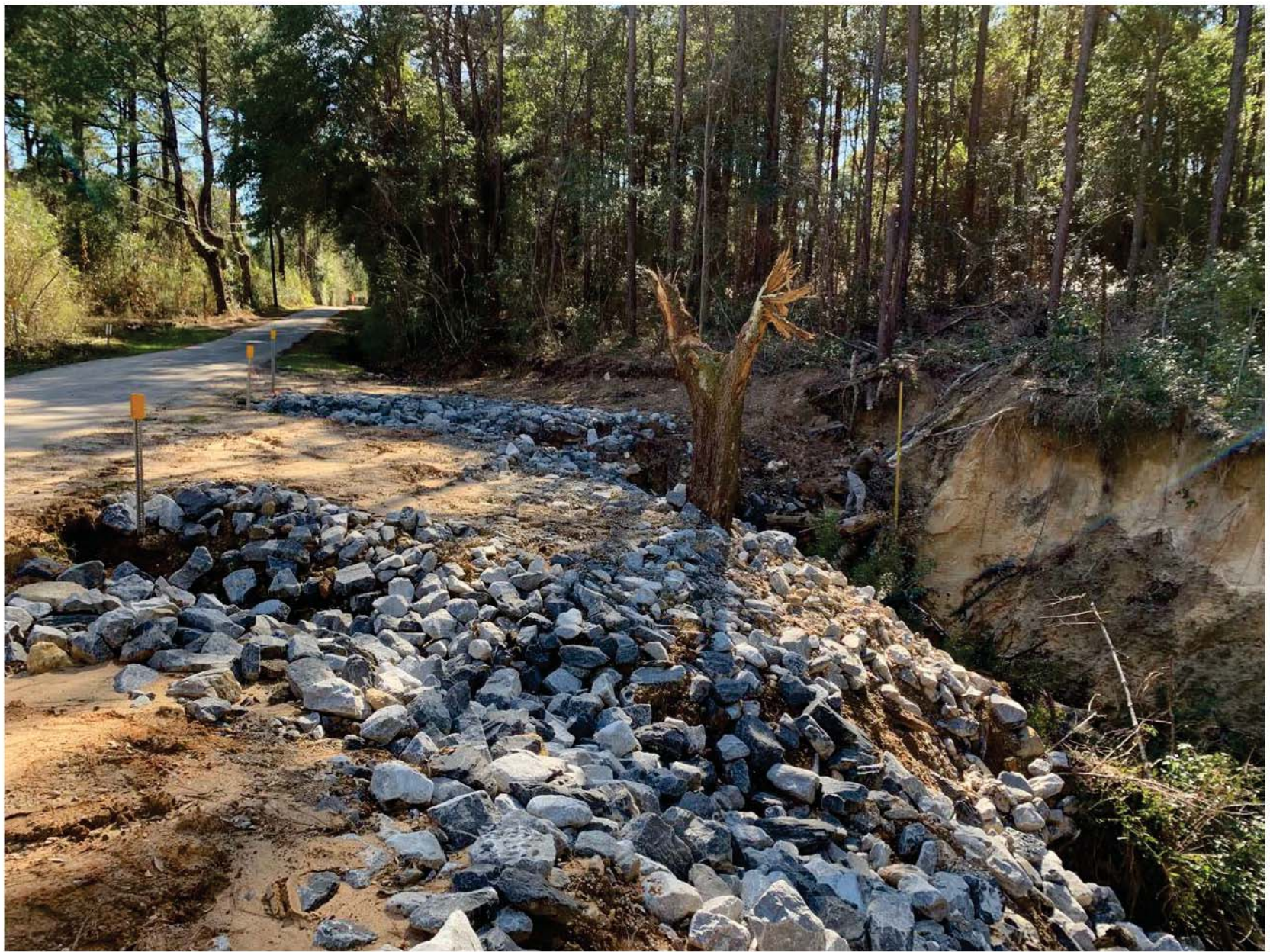
TURBERVILLE LANE 16' OF HEAD CUT AT ROAD
